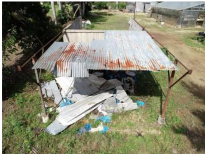
Soil Mixing Area
