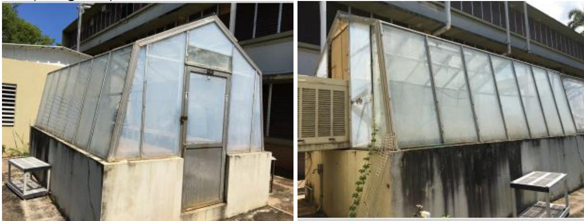
P023 Agricultural Greenhouse is a greenhouse that is constructed of metal framing situated on a concrete slab with a 3-foot concrete wall. The exterior consists of 2x6 plexiglass panels.
