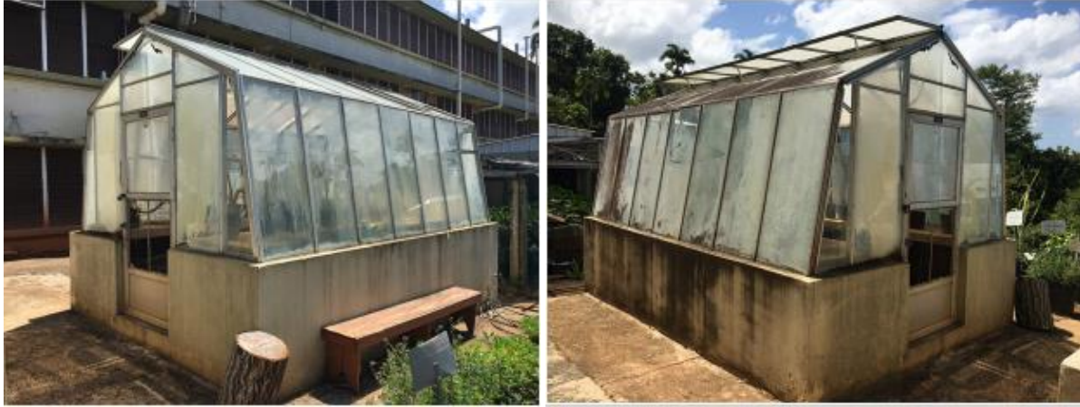
P023 Agricultural Greenhouse is a greenhouse that is constructed of metal framing situated on a concrete slab with a 3-foot concrete wall. The exterior consists of 2x6 plexiglass panels.
