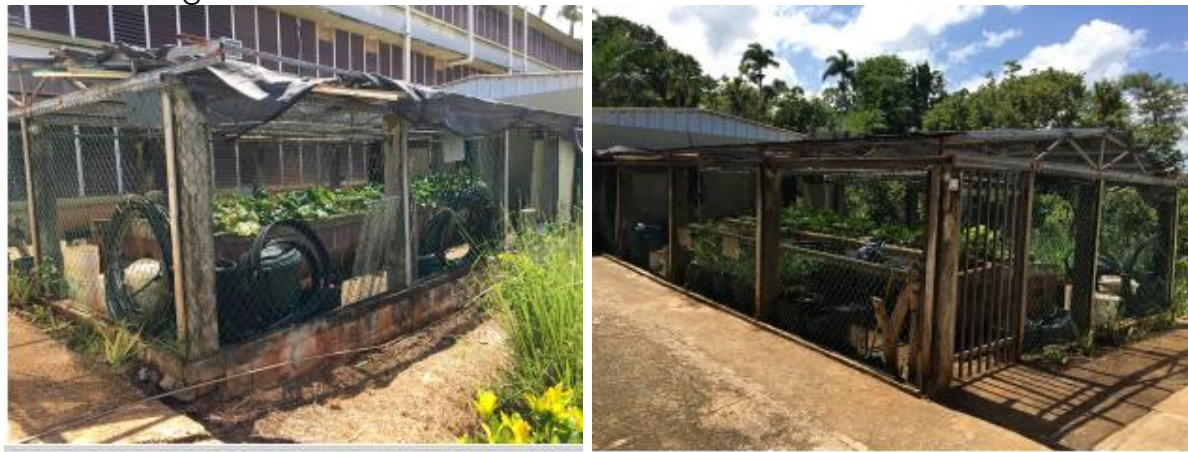
P026 Agricultural Greenhouse is a greenhouse that is constructed of metal and wood framing situated on 1-foot cinder block wall. The exterior consists of wire mesh fencing.
