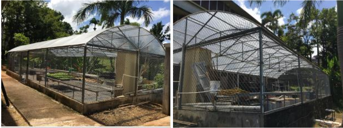
P026 Agricultural Greenhouse is a greenhouse that is constructed of metal and wood framing situated on 1-foot cinder block wall. The exterior consists of wire mesh fencing.
