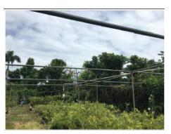
This facility consists of four greenhouses, Orchid Greenhouse, Vivero de Frutales Greenhouse, Introduccion Greenhouse, and Propagation Greenhouse. High winds, wind driven rain and flying debris tore up and blew off much of the PVC knitted windscreen causing the framework it was attached to deform, twist, and break. In additions other
